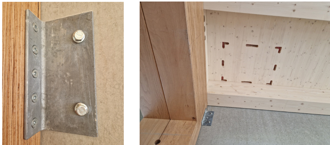
Fig. 7.2: Timber column to concrete connection with steel brackets and post-installed anchors at jobsite
