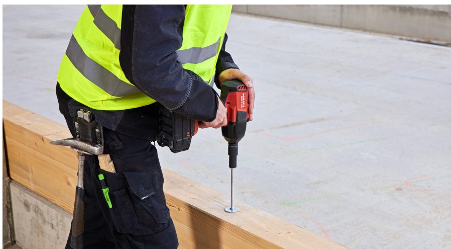
Fig. 2.3: Installation of a concrete screw anchor to fasten a timber beam to concrete directly through the timber element
