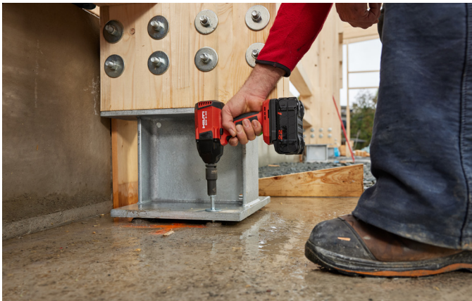
Fig. 2.5: Timber column to concrete application
