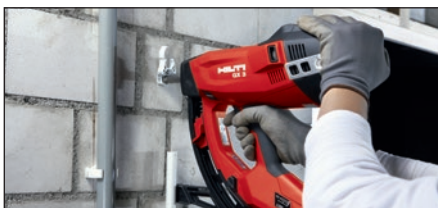
Conduits and light-duty pipes
