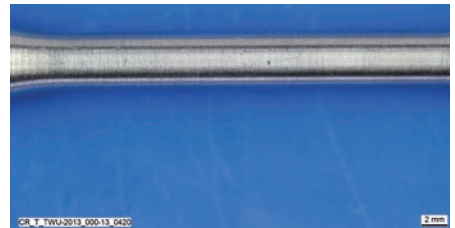
Suitable stainless steel used, e.g. HCR material used in a road tunnel
